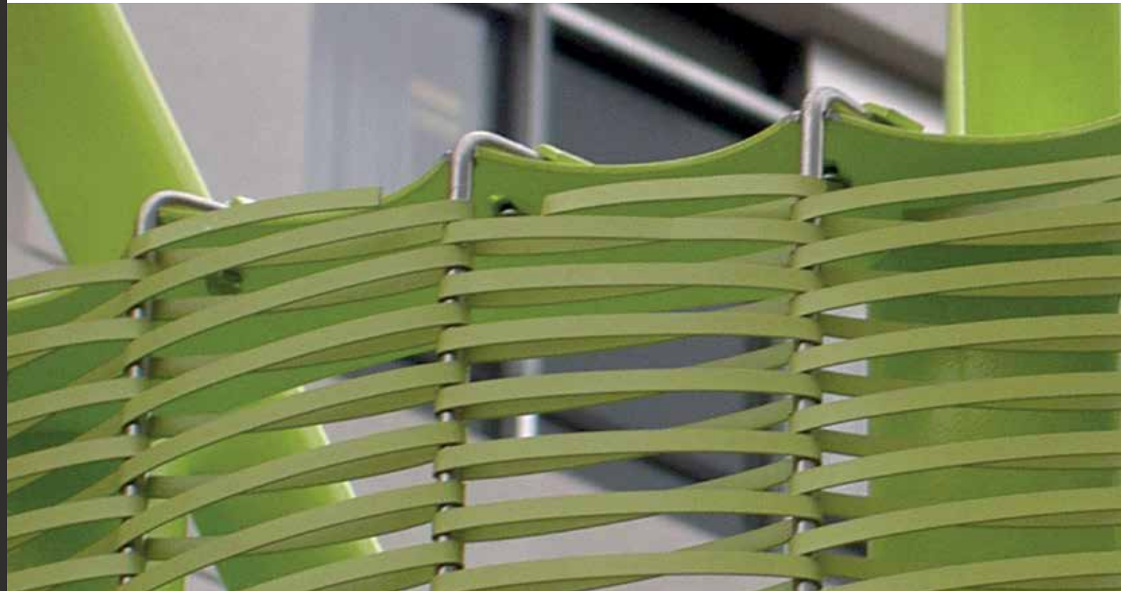
Mesh: Escale 7x1 painted green, project: St. Pölten orientation system, architect: Zieser
